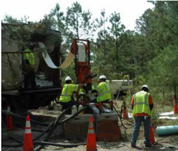
Sewer Repair at Cape Henlopen State Park
