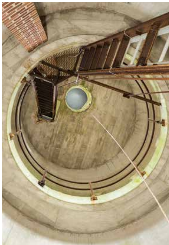
Tower 3 Interior Delaware Seashore State Park
