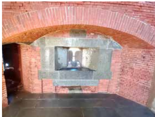
Fort Delaware Archway before and after repair
