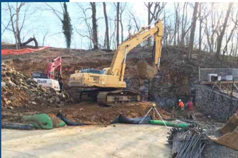
Construction of the Animal Support Building at Brandywine Zoo
