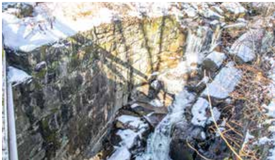
Stone Wall at Alapocas Run State Park
