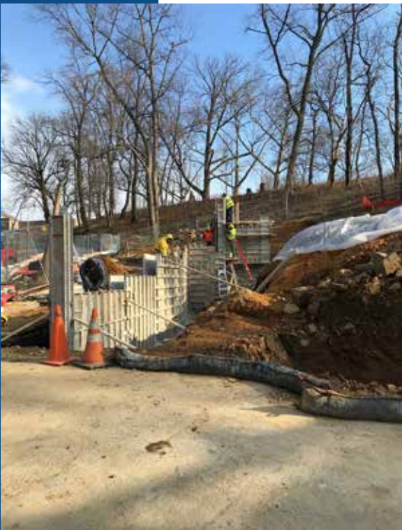
Construction of Brandywine Zoo Animal Support Building
