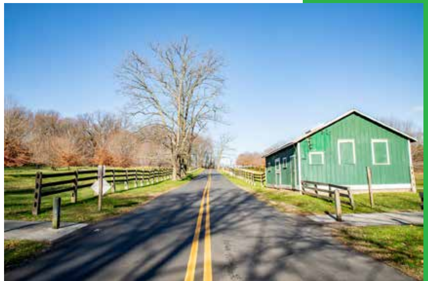
Bellevue State Park new pavement
