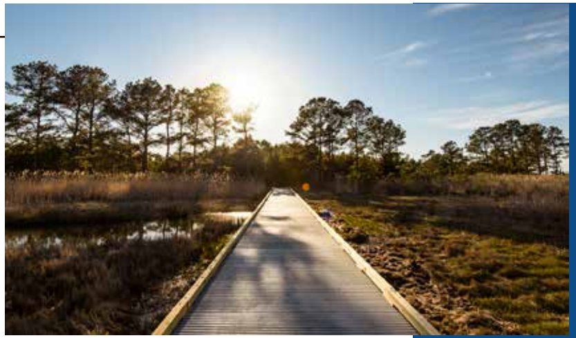
Sea Hawk Trail improvement at Holts Landing State Park
