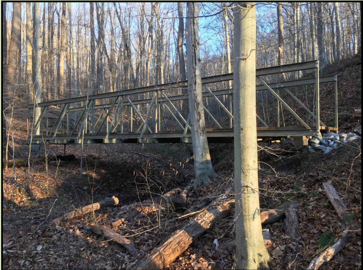
New Bridge on the Charles Bailey Trail
