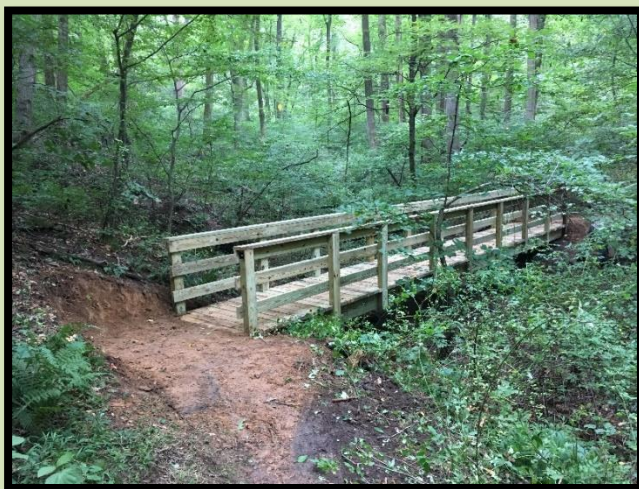
Typical Trail Bridge
