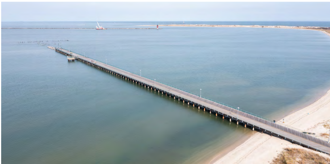
Existing Pier in need of replacement at Cape Henlopen State Park
