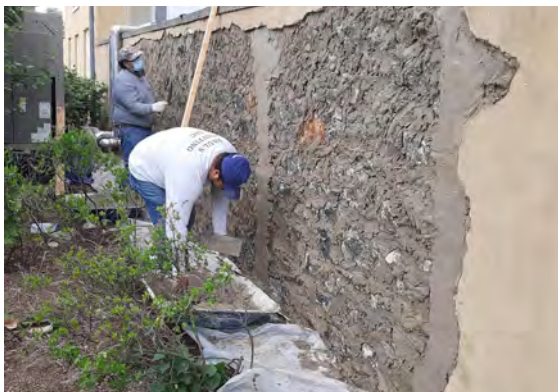
Repair of wall at Blue Ball Barn, Wilmington State Parks
