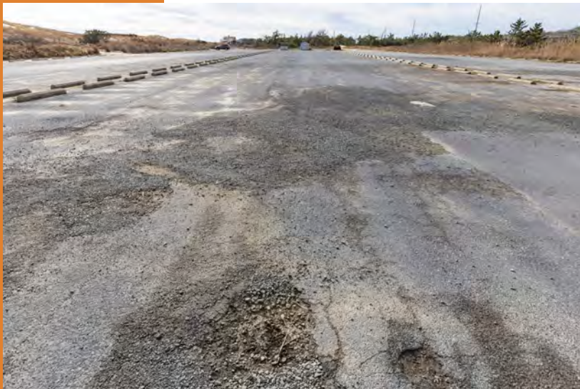
Parking lot at Fenwick Island State Park
