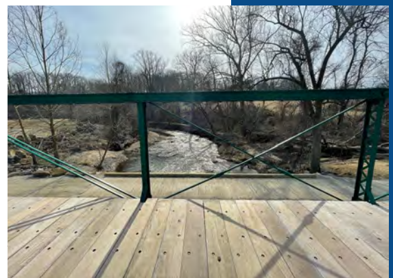
Farmlane Bridge at Auburn Valley State Park
