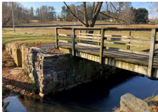
Wilson's Run Bridge
