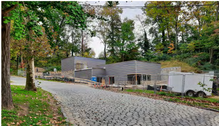
Construction of Brandywine Zoo Animal Support Building
