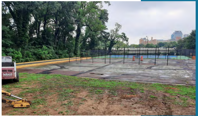
Lovering Avenue courts at Wilmington State Parks prior to renovation
