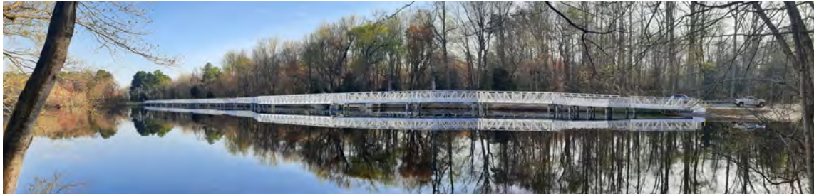
Elevated boardwalk at Killens Pond State Park
