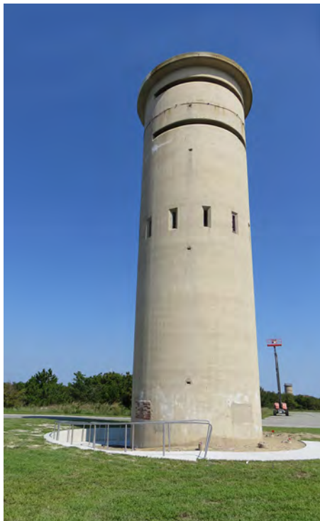
Restored Tower 3 at Delaware Seashore State Park
