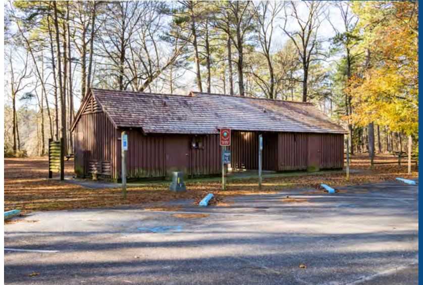
Bathroom at Cypress Point, Trap Pond State Park
