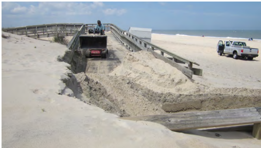
Boardwalk repair at Fenwick Island State Park
