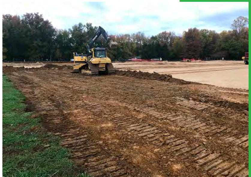
Lums Pond Recreation Area 1 Paving
