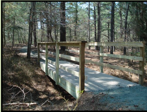
Typical Trail Bridge
